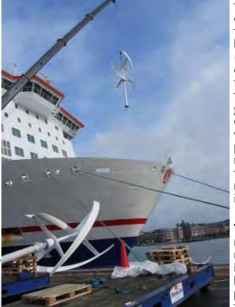
In June 2011, two UGE-4Ks were installed 4 meters above the bow of the Stena Jutlantica, a commuter ferry line Gothenburg, Sweden by Swedish distributor WindQ as part of Stena Line's environmental efforts. This is the world's first installation
