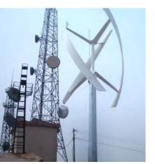
In July 2011, the Chinese Navy installed an **Urban Green Energy Fusion system** at a coastal location on mainland China to power one of their communication towers. The system consists of an off-grid **UGE-4K vertical axis wind turbine** with **2 kilowatts of solar.**
